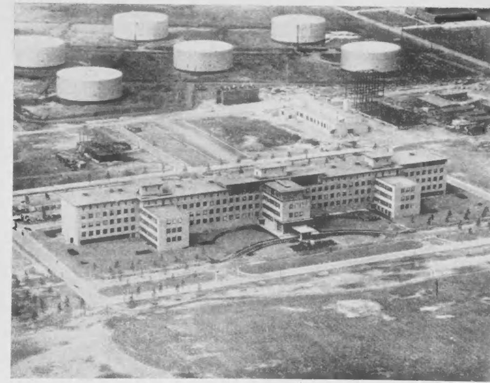
Shown above is the new Esso research center at Linden, New Jersey, which was officially opened on October 14. Built for the Standard Oil Development Company, the building is one of the most modern, as well as one of the largest, petroleum research centers in the world. The building above is the first unit of the center, and will house approximately six-hundred-and-fifty chemists, engineers, and research assistants. It has eighty laboratories, two-hundred-and-fifty offices, a technical library occupying the glass-enclosed center portion, an auditorium accommodating one-hundred-and-fifty persons, a lunchroom, and a sun deck located on the roof of the right wing. In the background are oil storage tanks of the Bayway refinery of the Esso Standard Oil Company.
